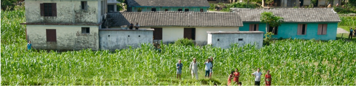
Figure M17. Masonry structures (200 m south of the liquefaction fissure) showed no evidence for damage except of the loss of a few tiles near end gables (Intensity 5-6).
